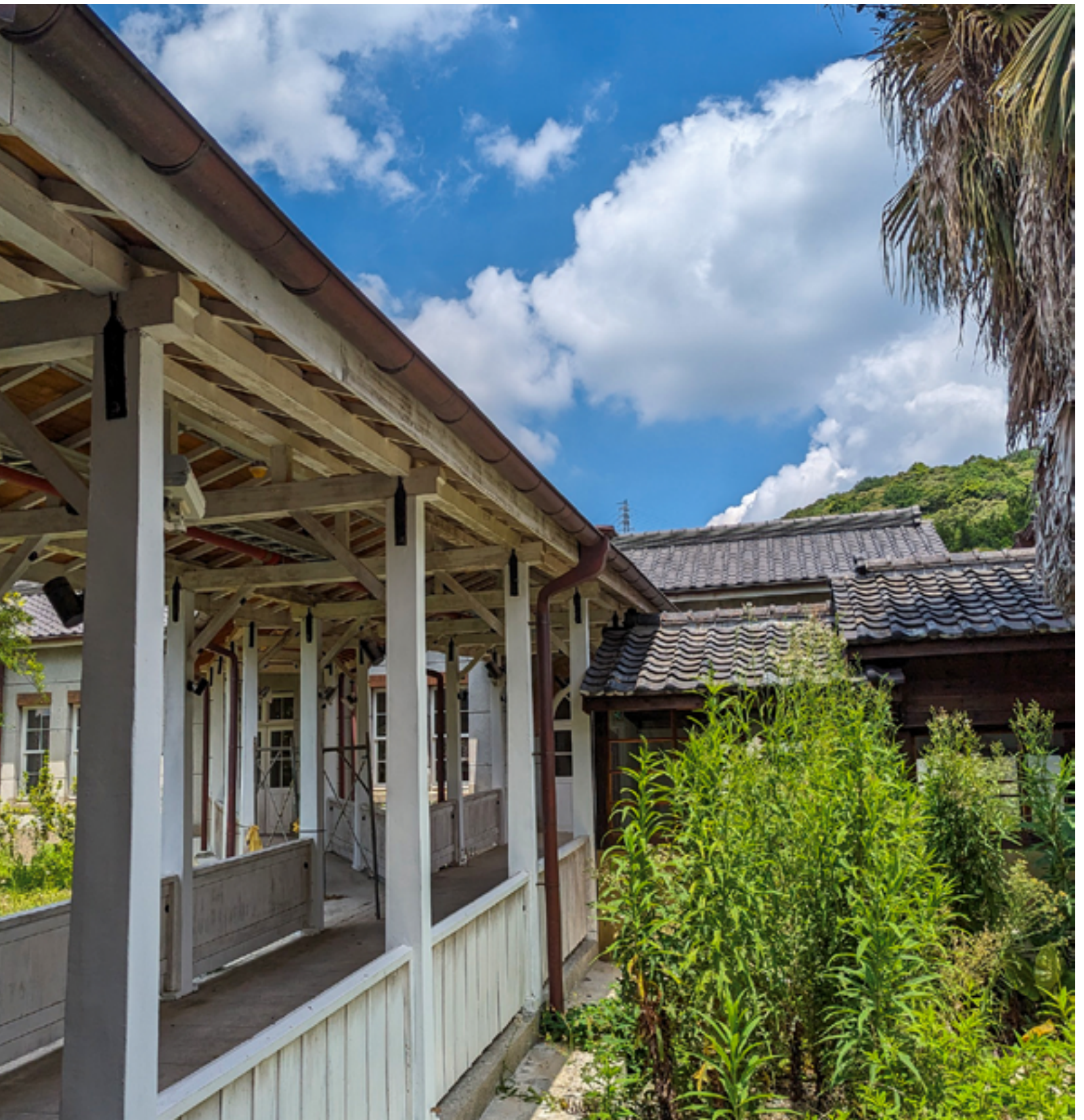
the connecting corridor at the Losheng Leprosarium built by the Japanese colonial government in 1930. Photo taken by Shu-Mei Huang in July 2023.
